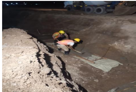
Gambar 4. 6 Pengecoran Lean Concrete
