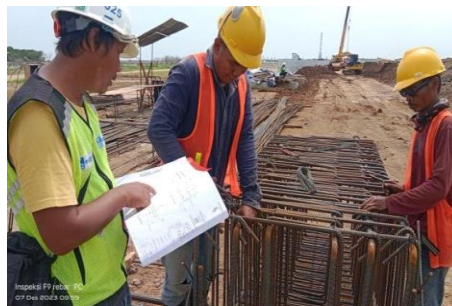
Gambar 4. 9 Pengecekan pembesian
