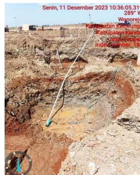
Gambar 4. 2 Proses Dewatering
